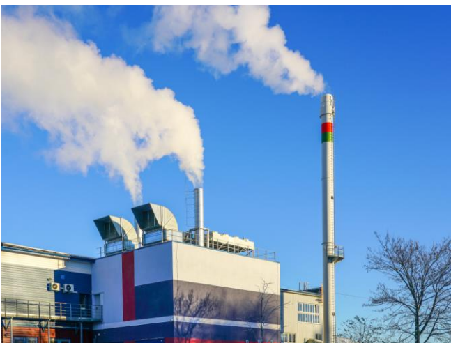
Combined Heat and Power Plant
