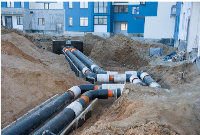
Repair of District Heating Network
